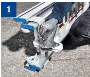
1 Mount the pulley and the winch on both support ladders, then thread in the ropes.
