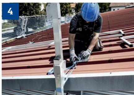
4 Anchor the posts with lashing straps.
