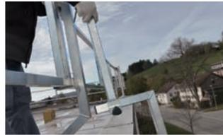
When wind rises and after work a parapet slip guard provides additional wind protection for the guardrail.
