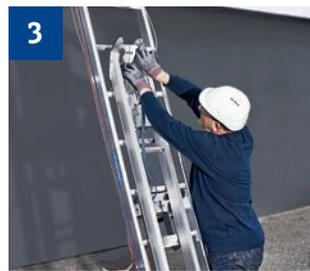
3 Attach the slides to the ladders and fasten the lifting ropes.
