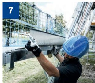
7 If necessary, install a bridging plate and toe board.
