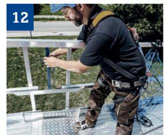
12 If necessary, join two platforms together using a connecting bridge.
