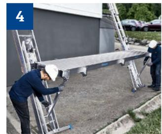
4 Attach the working platform and the connecting support to the slides.
