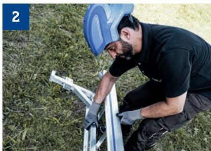
2 Attach the railing posts to the ladders.
