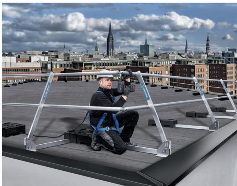
NEO 40 N assembly example with inclined post
