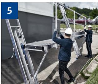
5 Insert the guardrail into the working platform and attach the safety net or rear guardrail, if required.
