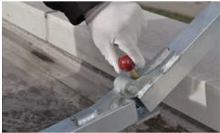
The cantilever can be folded up temporarily, which permits work in the cantilever area.
